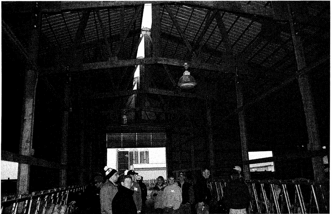
The reconstructed barn after installation of the proper rafters.
