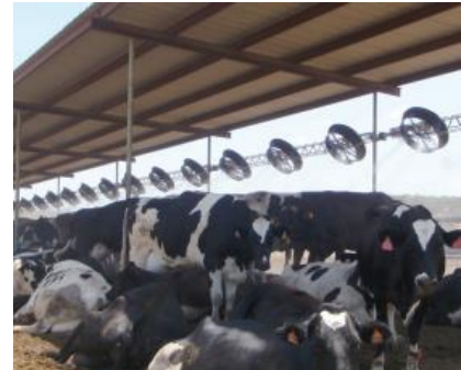
FIG. 3. FlipFan system cooling cows under a dry-lot shade.
